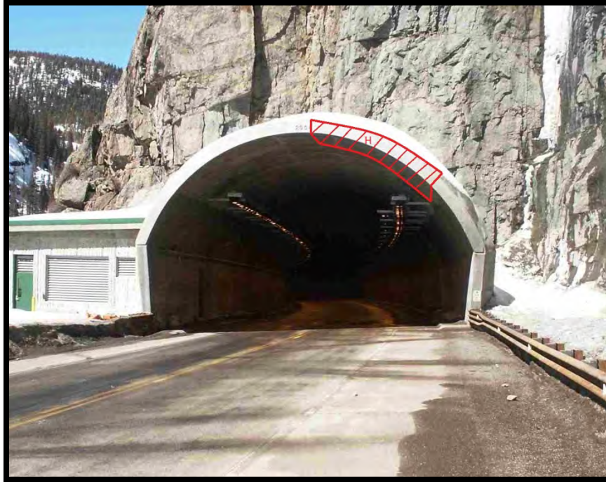
Photo 1: Example - North portal, looking south
